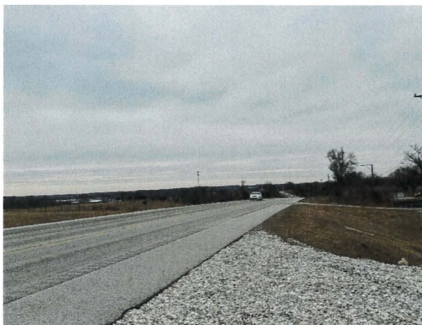
View North of State Road 135 (South Main Street)
